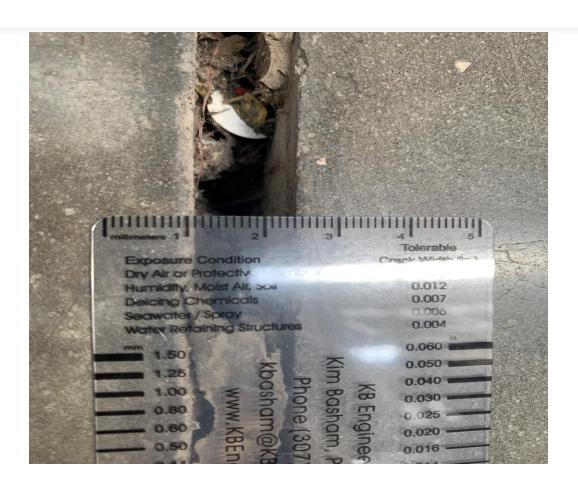
Widening of joints within one year after construction is normal behaviour. Initially, joints are sealed with soft and elastomeric sealant, which ultimately gets debond or split with time. Therefore, re-sealing of joints with appropriate sealant is important which maintains the balance between joint opening and hardness of the sealant.
